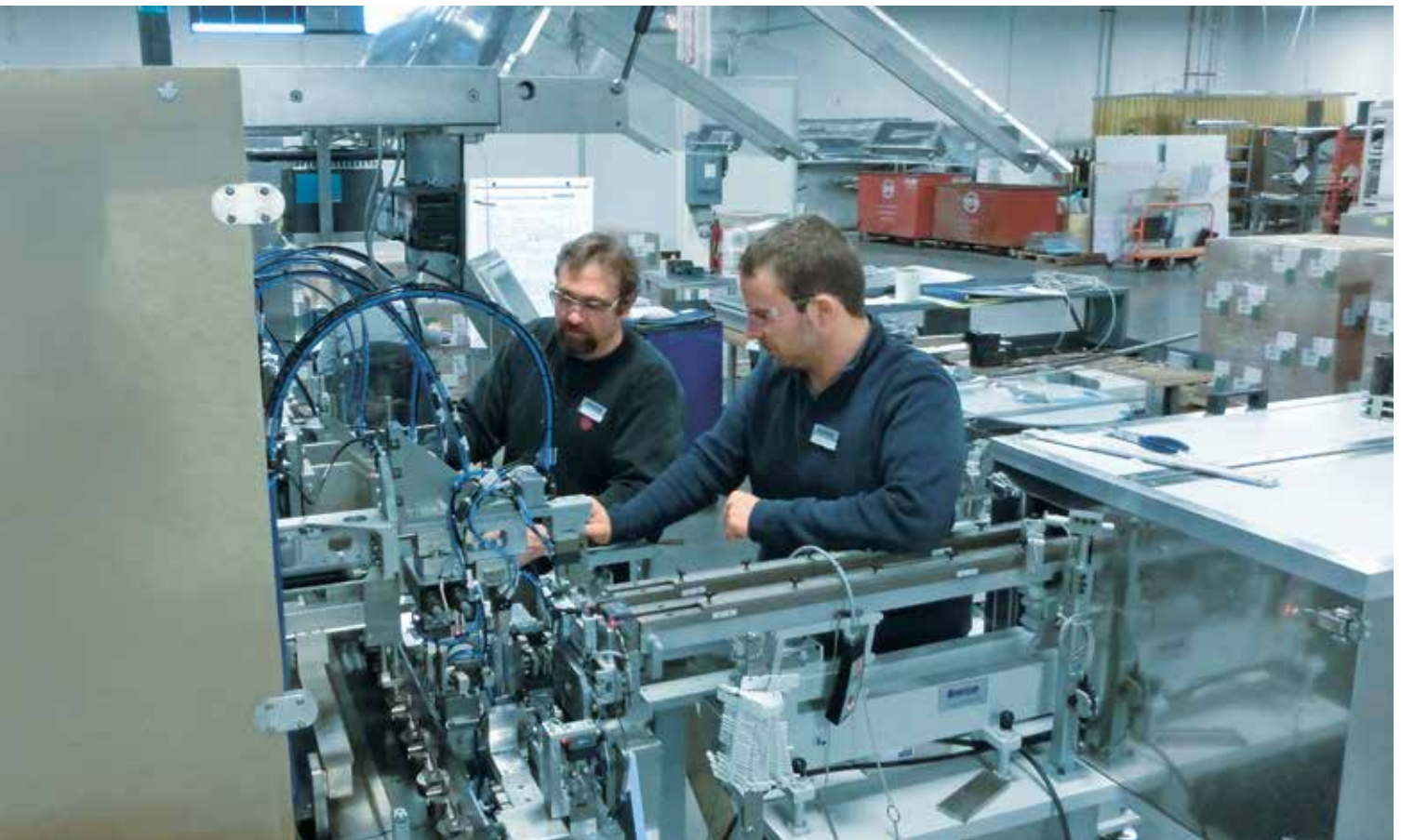
The team in Denver managed the project and installed the complete solution.
